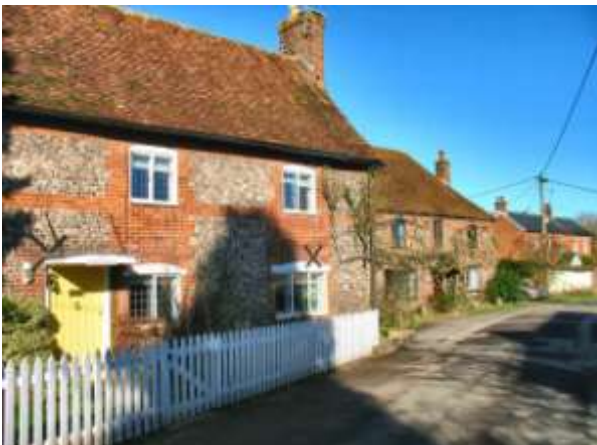
Photo 27: The Dairy House, High Street, Porton - built of brick & flint and roofed in plain tiles
