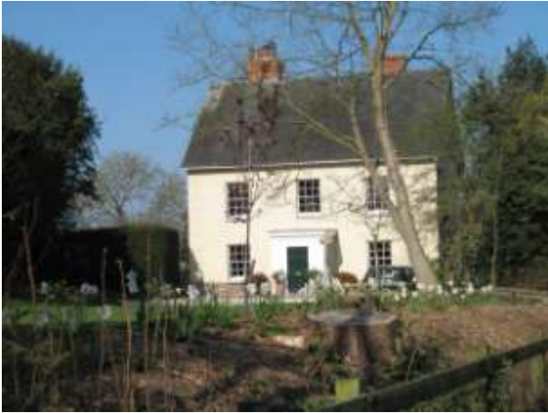
Photo 26: Chalk House, Porton – a landmark building of colour-washed cob under a slate roof
