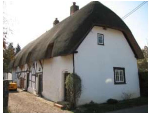
Photo 28: Ti Tree Cottage, High St, Porton - timber framed cottage extended in flint/cob under thatch
