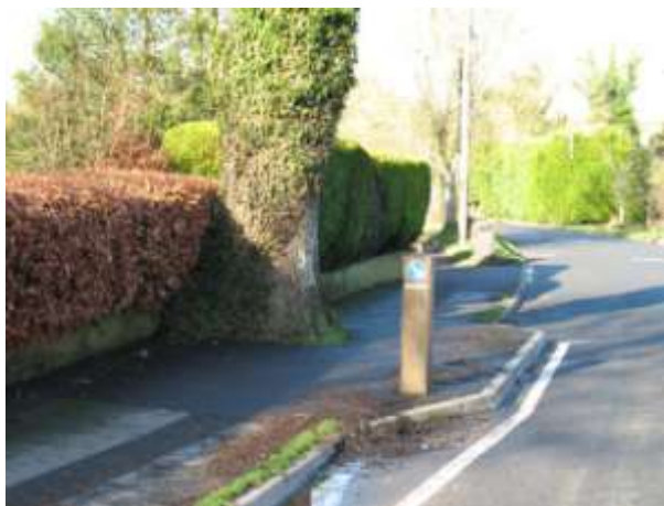
Photo 44: Winterslow Road pavement build out
