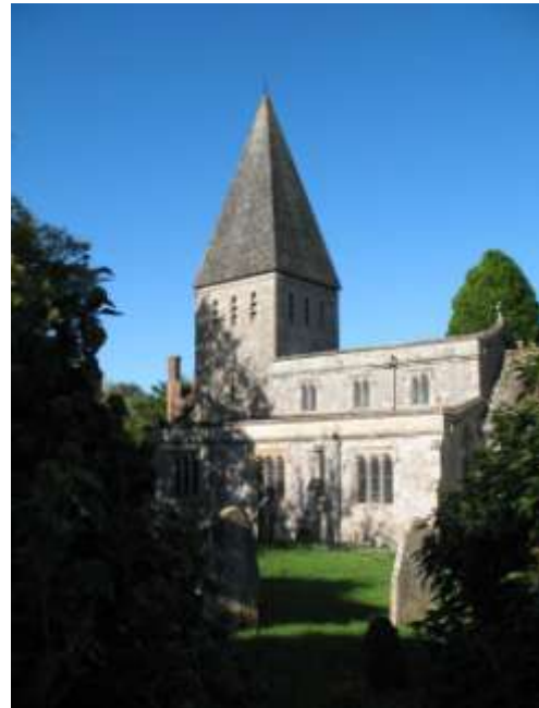
Photo 25: All Saints Church, Idmiston - constructed of flint with limestone dressings
