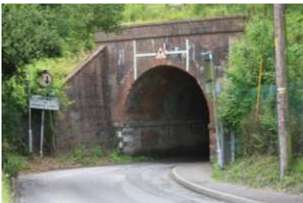
Photo 46: Gomeldon Rail Bridge – a bottleneck in the morning rush hour
